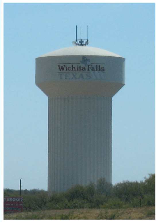
Exisiting Water Tower
